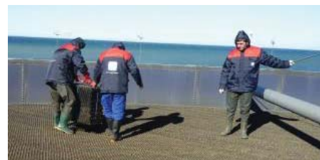
Fig.2: Media check at trickling filter in Batumi (Georgia)
